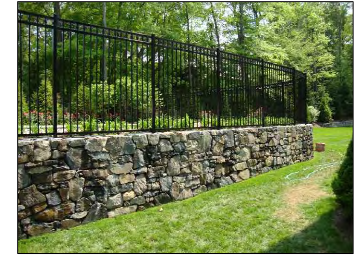
BLACK METAL RAILING WITH STONE COLUMNS
